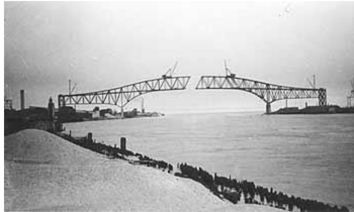
Blue Water Bridge under construction, circa 1938. Source: MDOT
